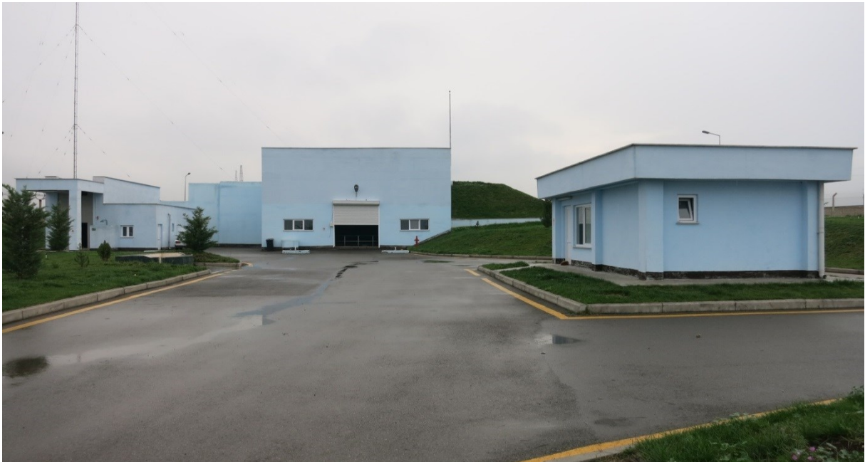
Newly constructed water reservoirs for water distribution to different parts of Shaki.
