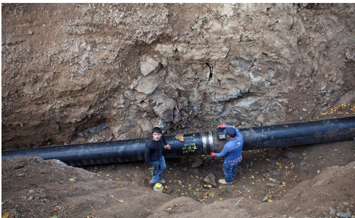
Construction of a water pipeline near Ganja city.
