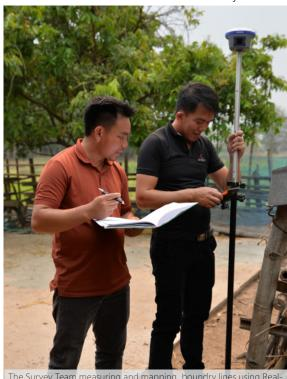
The Survey Team measuring and mapping boundry lines using Real-Time Kinematic satellites. © SDC/Toula HOOK
