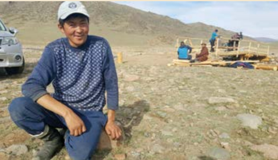
D. Dugersuren and his friends building a bridge. © SDC
