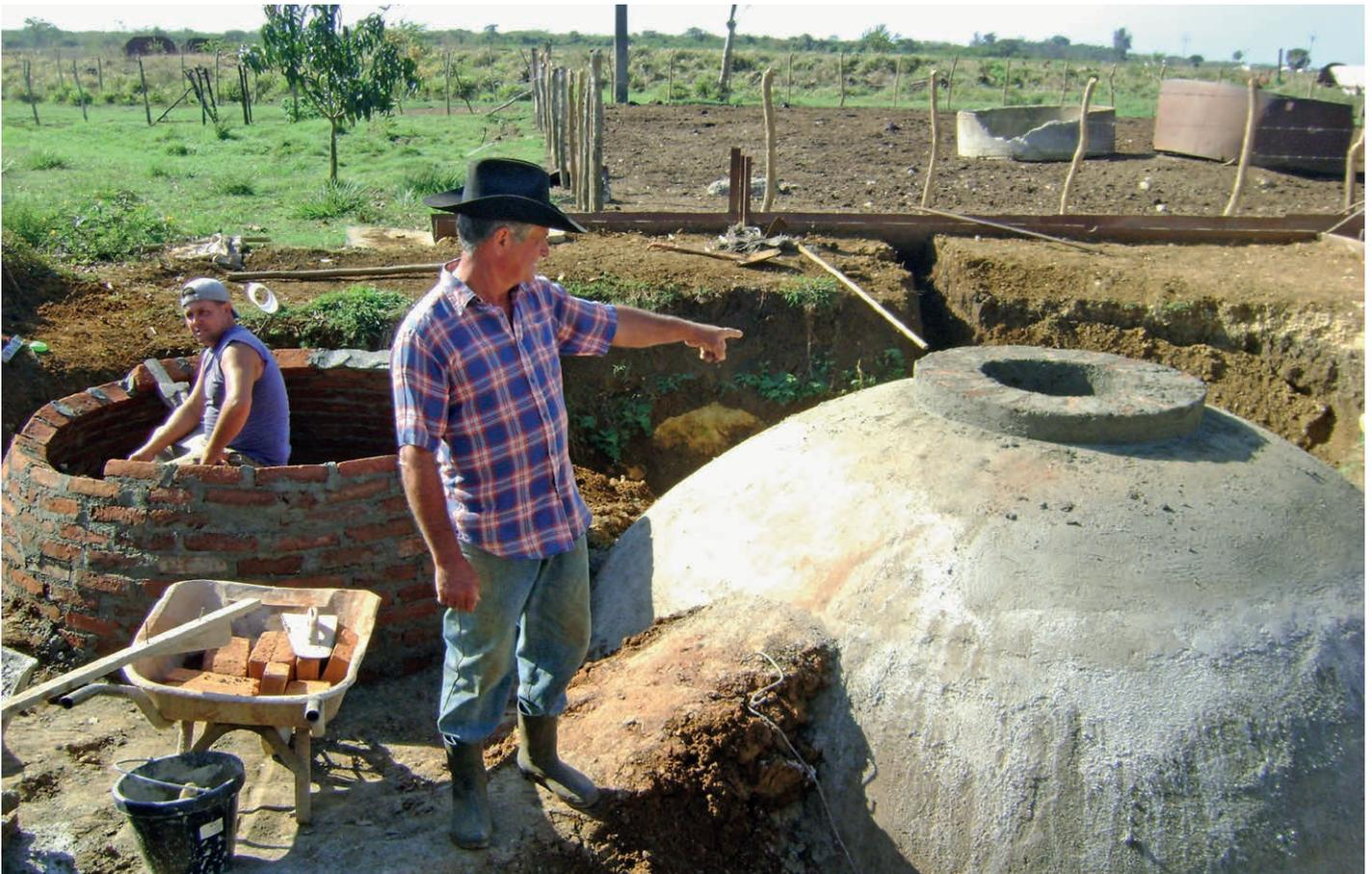
Cuban smallholder farmers take advantage of biogas plants to dispose of their pig slurry and generate gas for their own use
