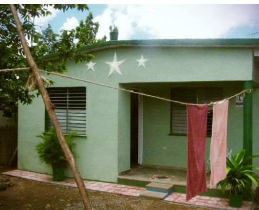
A house recently constructed using local resources within the framework of the PRODEL project, Aguada de Pasajeros.
