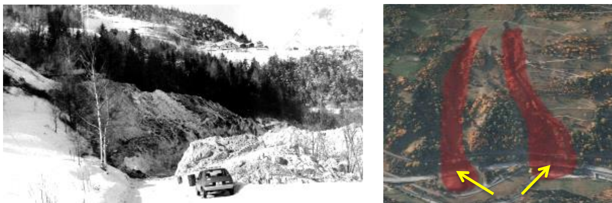
Figure 8, left: Snow deposits on the road after the avalanche of 1981. Right: The two avalanche paths (yellow arrows pointing to the two galleries).
