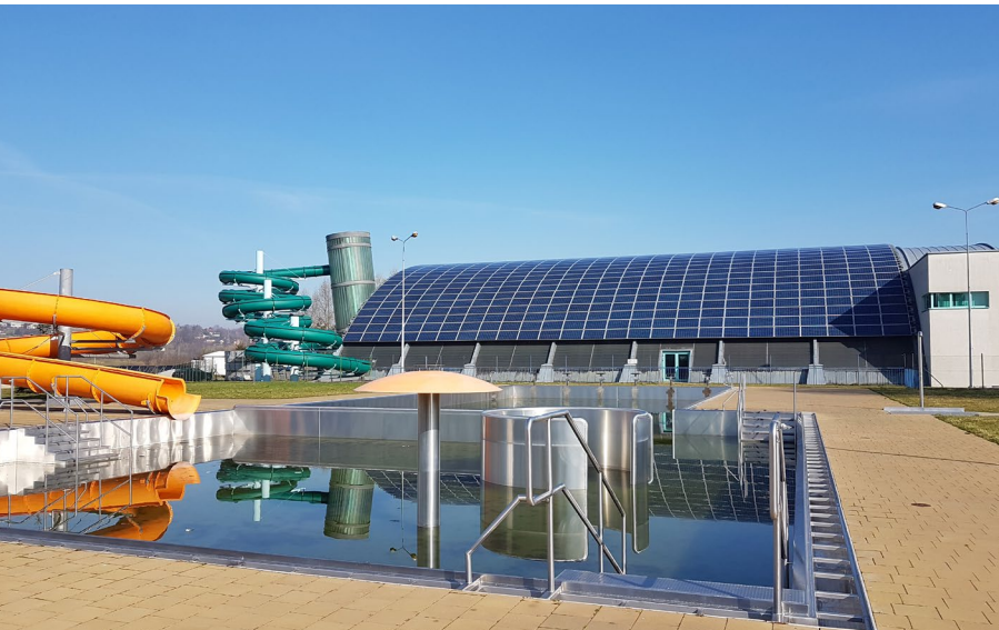
The roof of the swimming pool in Jasło, north-east Poland, has been covered with solar panels. © Local authority association of Wisłoka river basin
